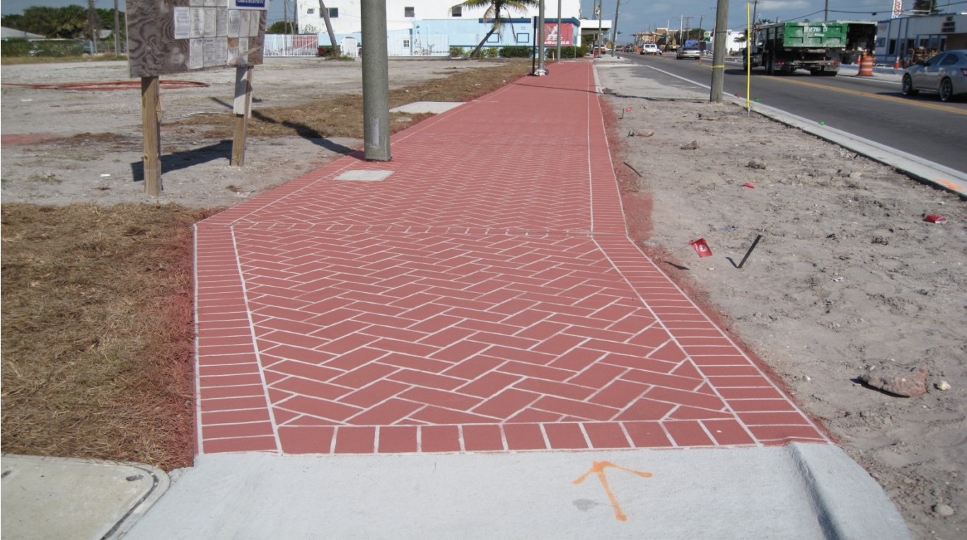
CITYBRICK ( FDOT SPEC # 523-0017) Slip resistant Patterned Sidewalks
